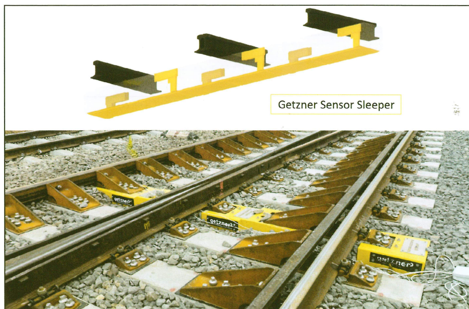
Fig. 14: Equipped demonstrator sleeper of the Shift2Rail project
